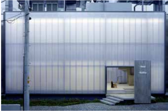
polycarbonate external cladding to extended cores
